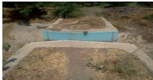
Fig.no.3Acut-throat flume
