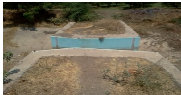
Fig.no.3Acut-throat flume
