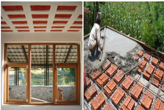
Figure 4 Casting of Filler Slab
