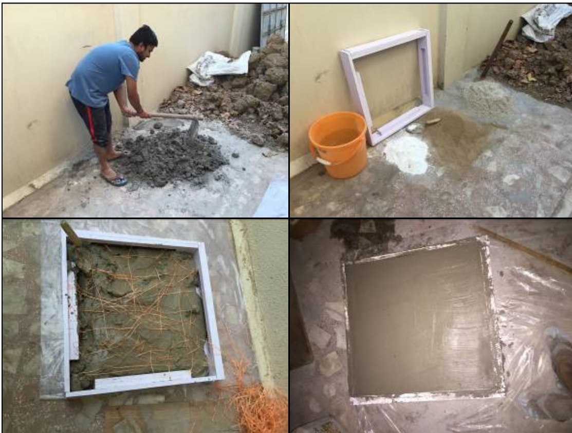
Figure: - Mortar casting
