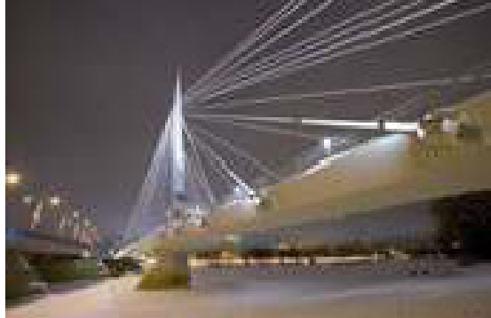
Fig1: Side-spar cable-stayed bridge, Esplanade Riel, Winnipeg, Manitoba .
