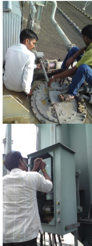
Fig.2: Troubleshooting of OLTC broken rod of 100MVA transformer by the BDM committee workers (left), and manually operating the tap changer (right), at 220/110kV R/S Vajjarmatti, Mudhol Tq. Bagalkot.
