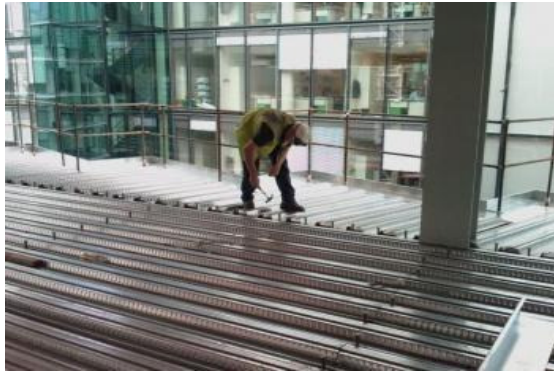
Fig. 1 Composite deck slab
